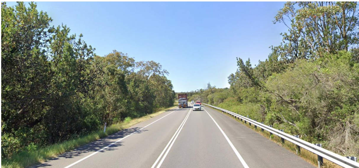
Figure 2.6: Nelson Bay Road Facing South
